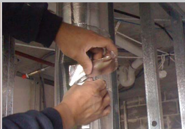
Simply use AGC tape to affix and join Soundlag even around complex bends in pipework.
