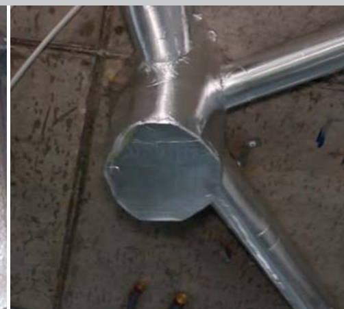
Simply use AGC tape to affix and join Soundlag even around complex bends in pipework.
